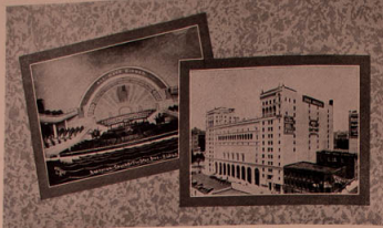
Interior of the Addition. Main Building Bible Institute.
